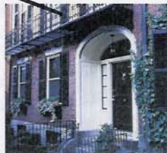
Entry details - planters, red iron and balconies
