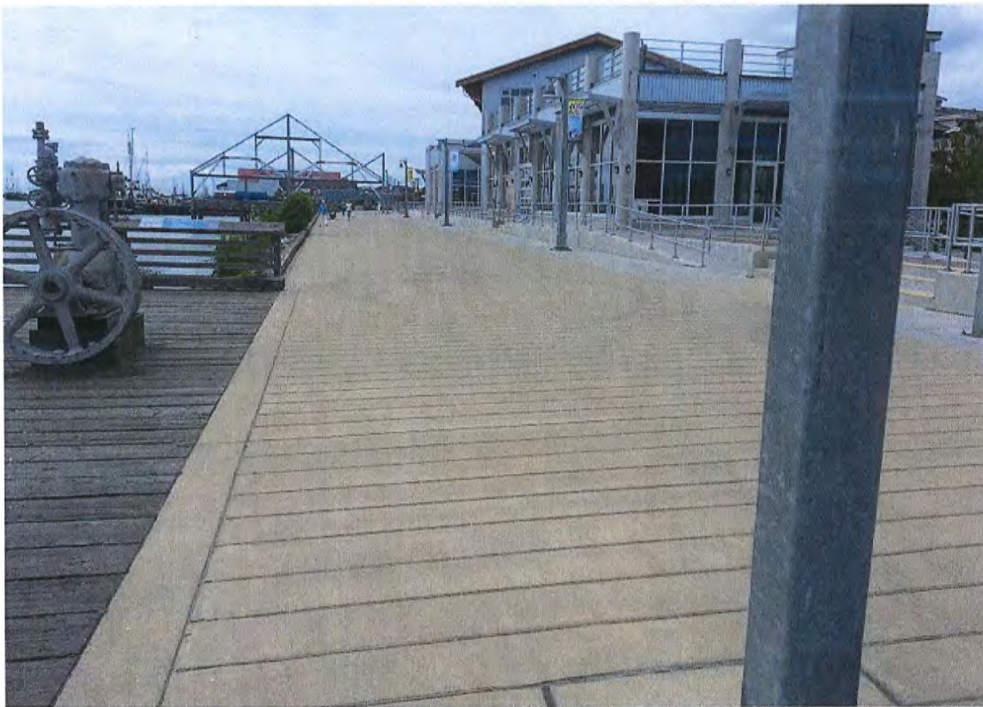
Concrete Textured to Appear as Wood Planks: Waterfront Boardwalk Parallel to Bayview Street East of No. 1 Road
