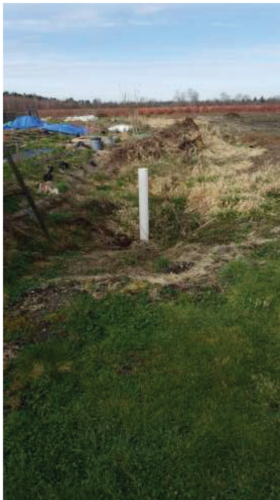
Figure 5 Surface Inlet to storm drain (looking west along southern parcel boundary at SW corner of Lawn area
