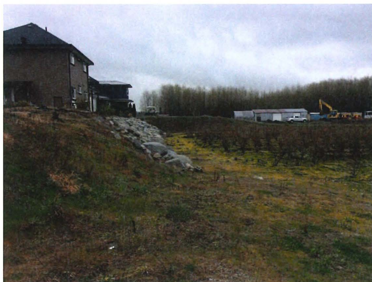
PHOTO 3. LOOKING EAST WHERE THE BLUEBERRY FIELD (NATURAL GRADE OF THE LAND) MEETS THE BERM (COMPACTED BOULDERS) CONSTRUCTED TO RAISE THE RESIDENCE TO THE FLOOD CONSTRUCTION LEVEL (3.5 M GSC). The residence is on the top left of the photo.
