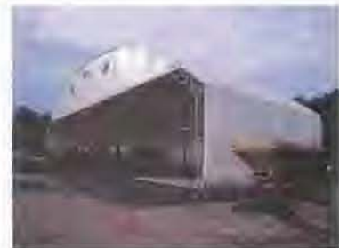
Figure 1: Snow shed located at Public Works Yard
