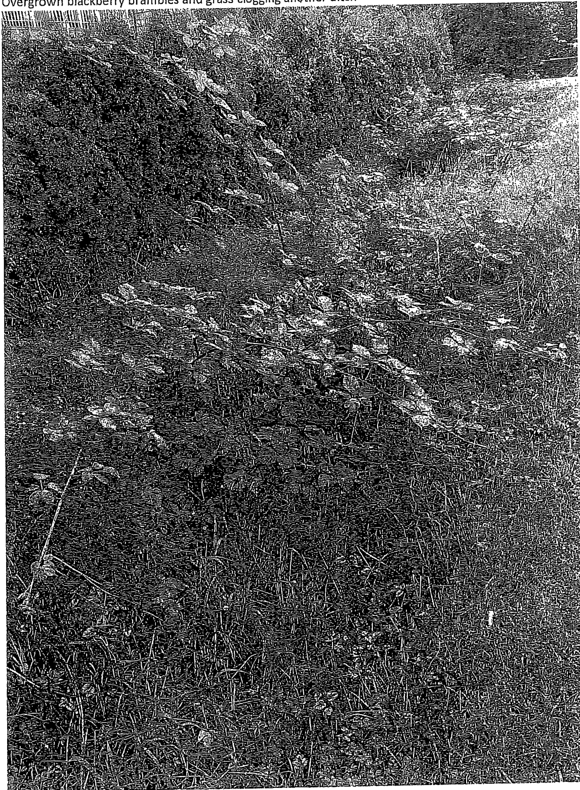
Overgrown blackberry brambles and grass clogging another ditch
