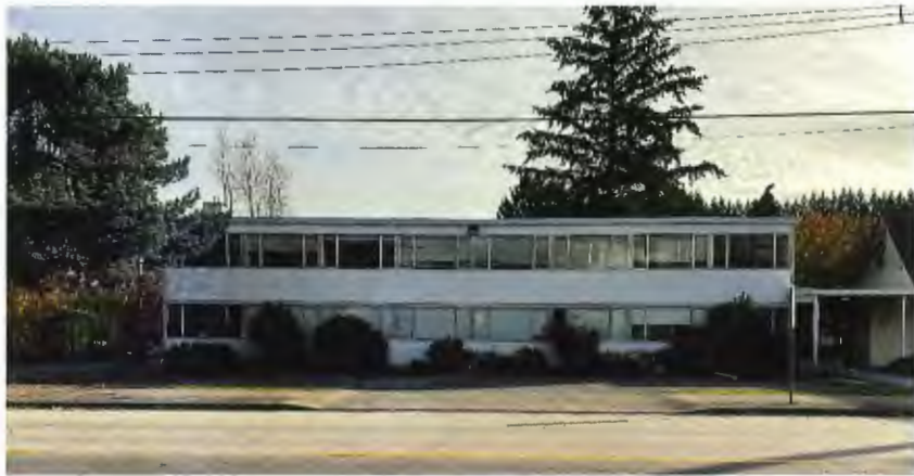
Church - flat roof
