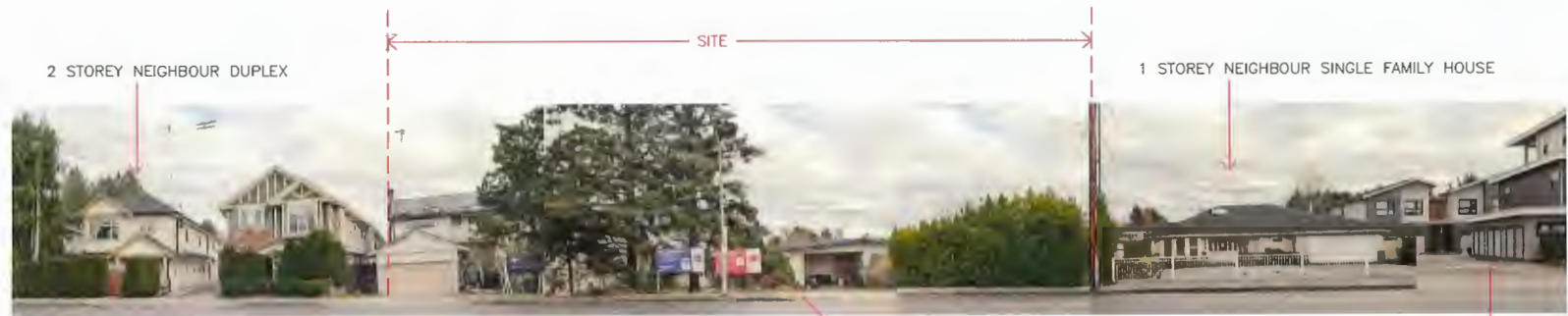
SITE VIEW FROM NO 1 ROAD
