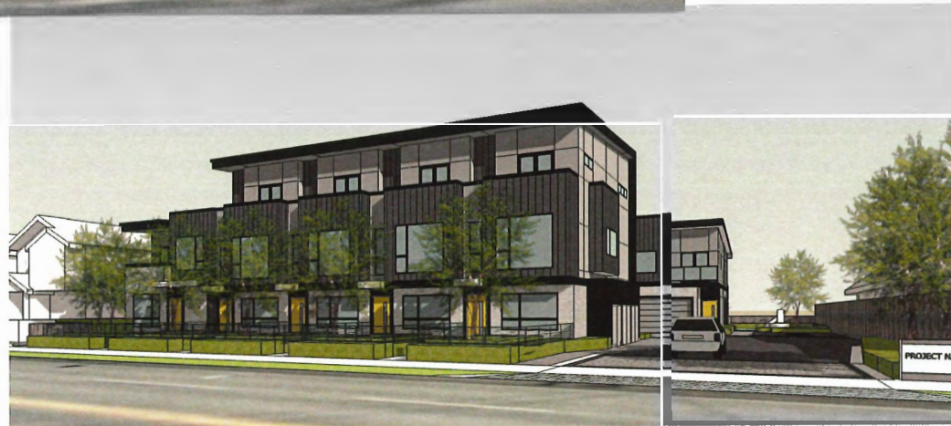
VIEW FROM NO. 1 ROAD
