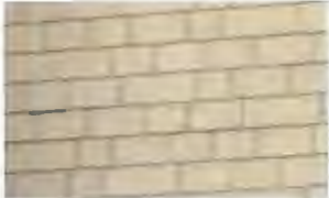
WALLS/BOX OUT: HARDIE SHINGLES
