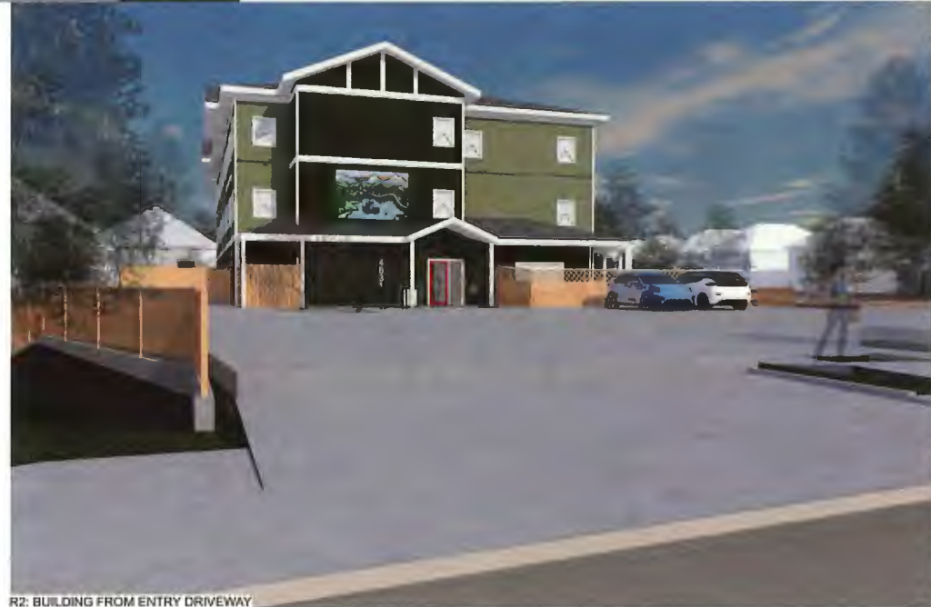
R2: BUILDING FROM ENTRY DRIVEWAY
