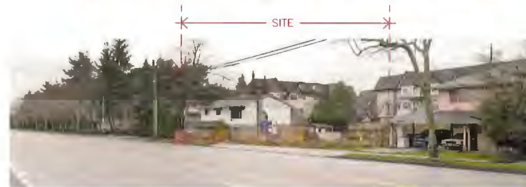
SITE VIEW ACROSS NO 1 ROAD
