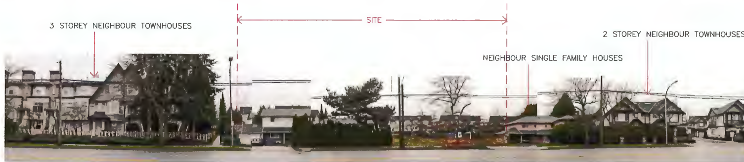
SITE VIEW FROM NO. 1 ROAD
