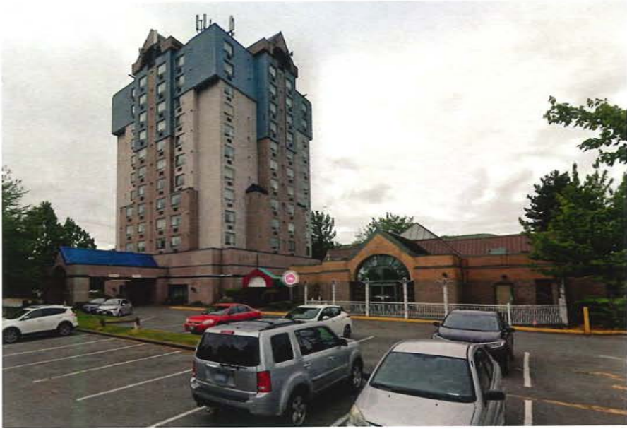
PICTURE OF EXISTING BUILDING
