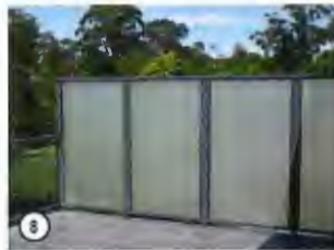
8 FROSTED GLASS PRIVACY SCREEN BETWEEN BALCONIES
