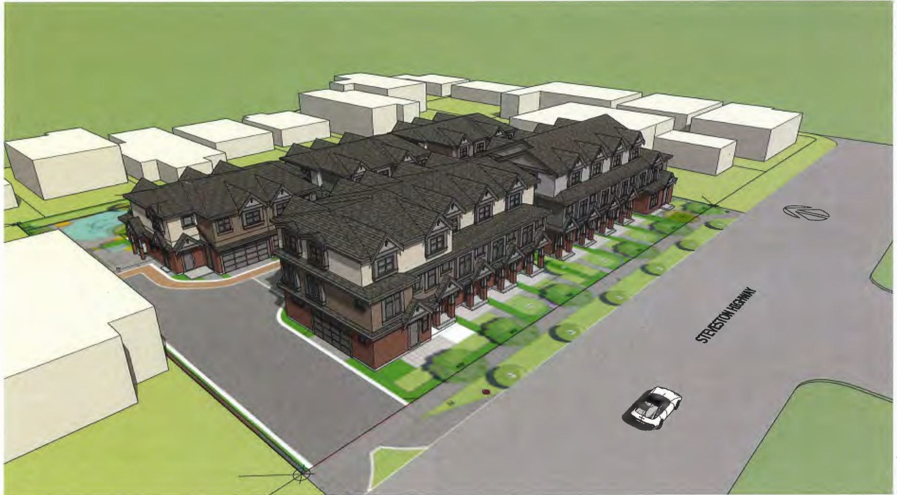
16 UNIT TOWNHOUSE DEVELOPMENT (DP 20-919145) AT 4571, 4591, 4611 STEVESTON HIGHWAY, RICHMOND, BC ISSUED DDP REVIEW 2024-01-17
