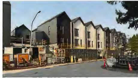
F THREE-STOREY TOWNHOUSES UNDER CONSTRUCTION
