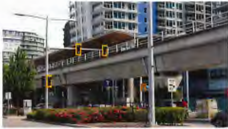
A RICHMOND - BRIGHOUSE SKYTRAIN STATION
