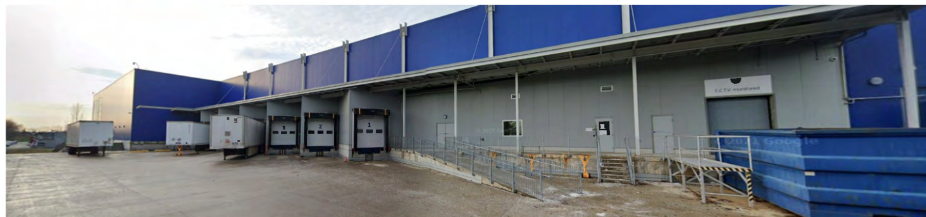
3 Existing West Loading Area View (Photos taken from Google Earth)
