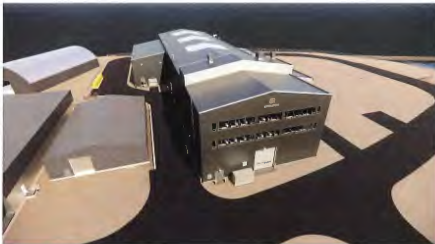
New machine shop showing attached welding/fabrication shop
