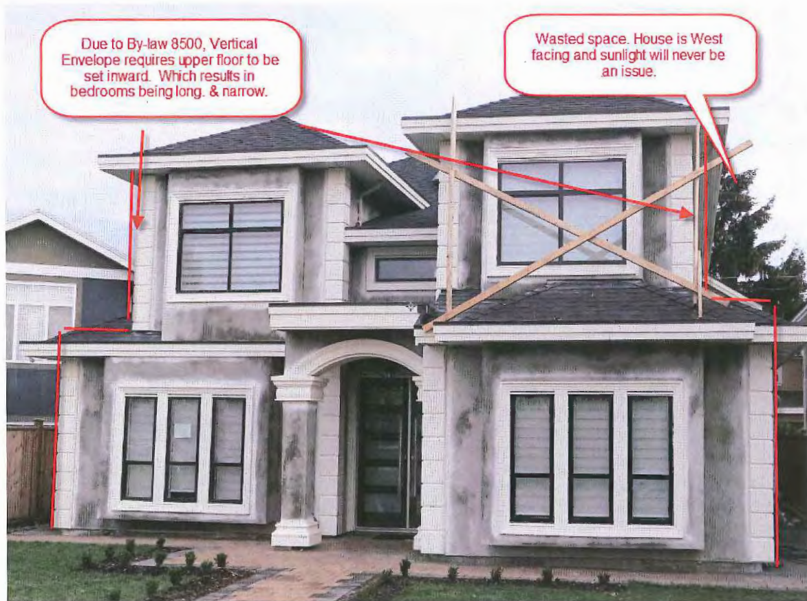
Figure 12: Unnecessary forcing of upper floor for privacy & sunlight
