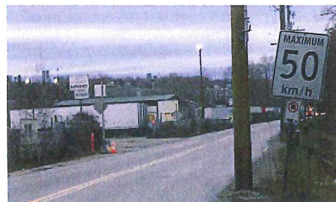
River Road Looking East (near No. 6 Road). Utility pole close to edge of road.
