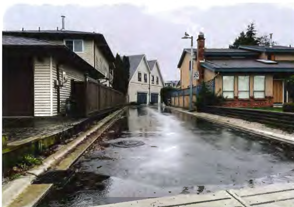
Fig.4-Partially upgraded portion of the laneway with lighting, speed signage, curbing, and drainage improvements.
