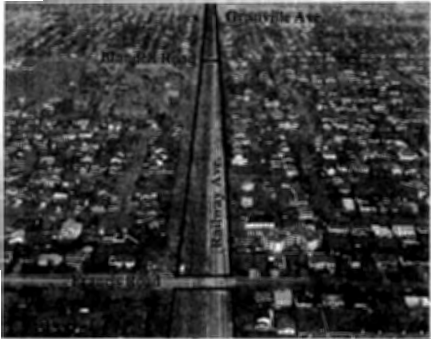
Aerial photograph looking north from Francis Road to Granville Avenue
