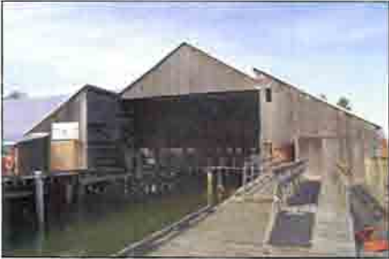
Slipway at the Britannia Heritage Shipyard (c. 1889-1890)
