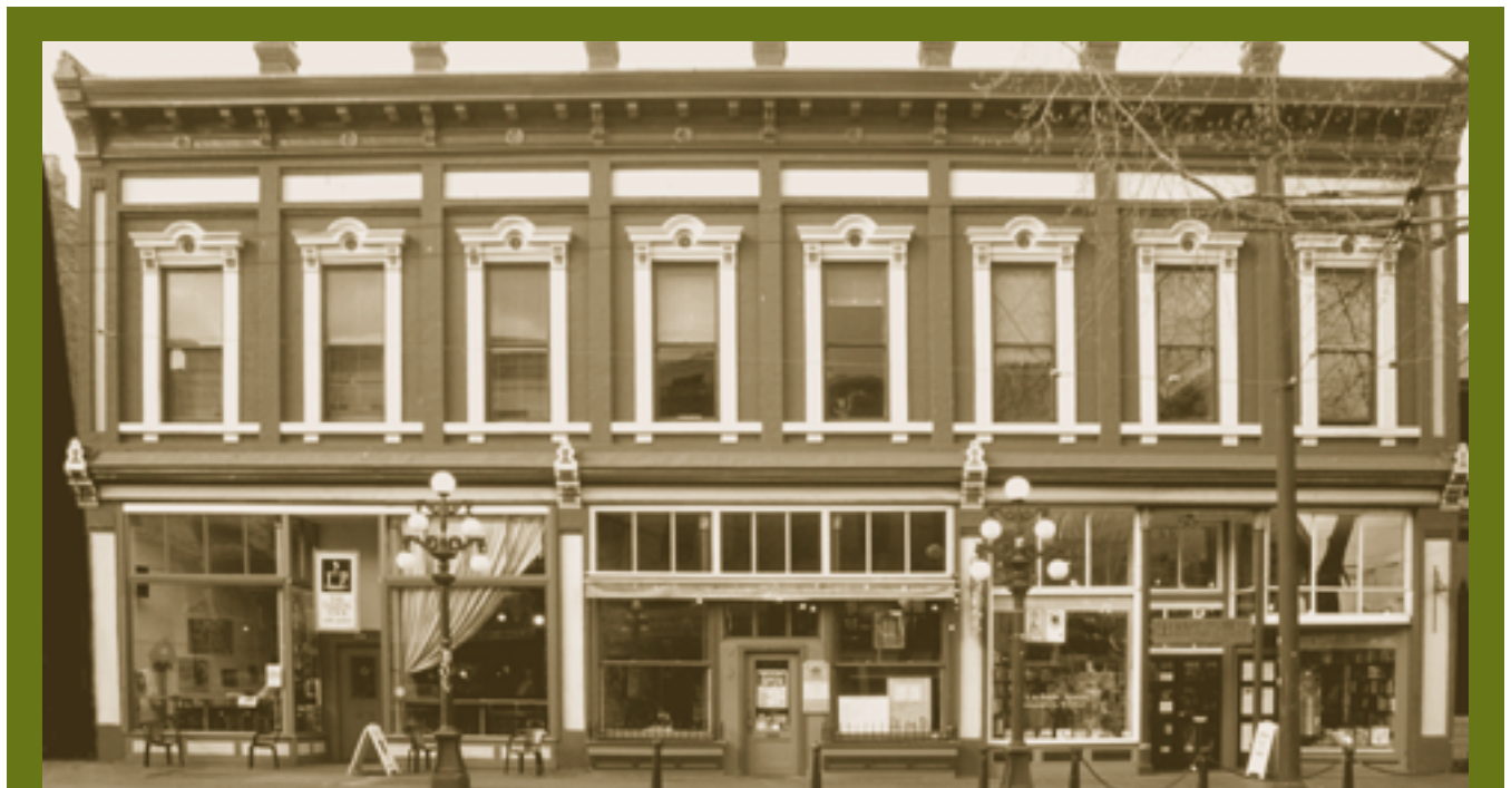
The character-defining form and features of 1880s storefronts in Vancouver, including their large plate-glass display windows with multi-pane transom windows above and recessed central doorways, have been retained through Preservation .
