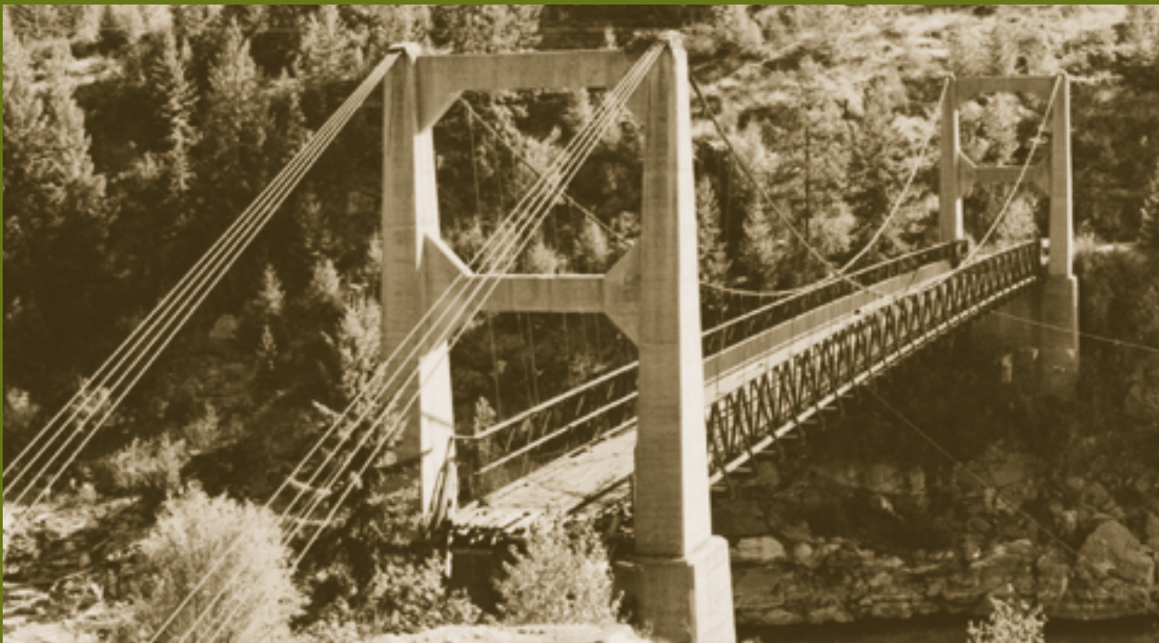
The Brilliant Suspension Bridge was built over the Kootenay River near Castlegar, British Columbia in 1913. Ensuring public safety is one of the primary concerns of professional engineers.
