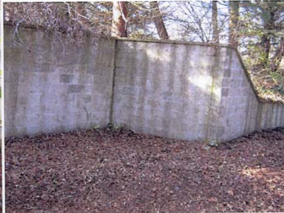
Retaining walls in the “Secret & Contemplative Garden” are in good condition with some small patch repairs needed.
