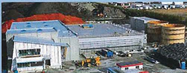
Harvest Power's new anaerobic digester under construction.
