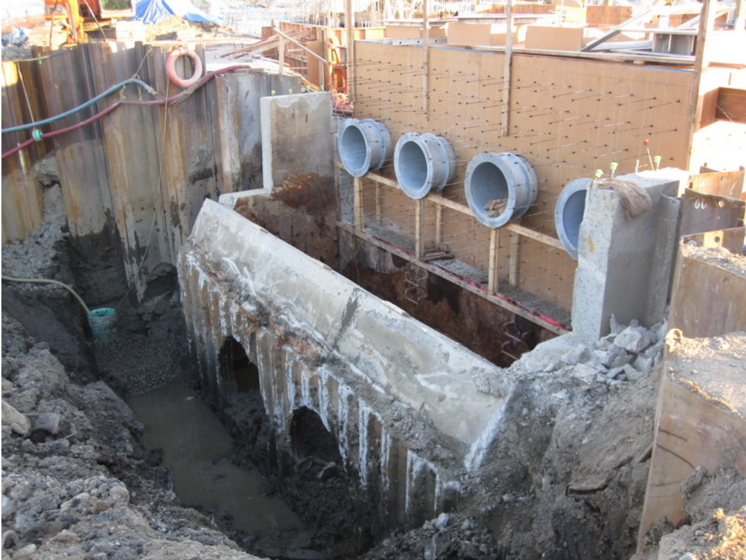
Flood Box Demolition/Construction
