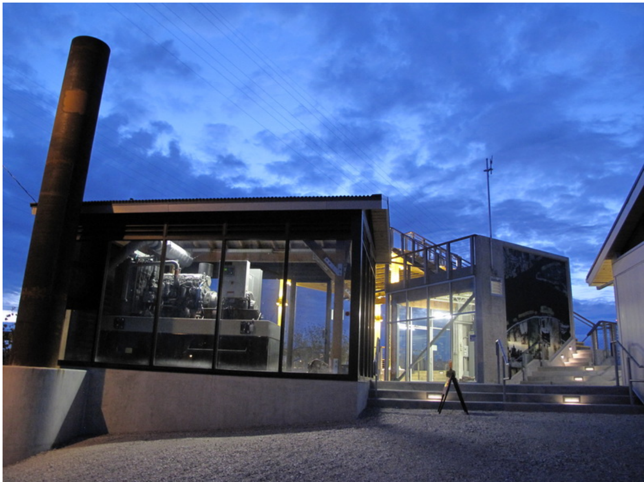
Completed Pump Station- Back-up Generator Building (Left) and Control Building (Right)
