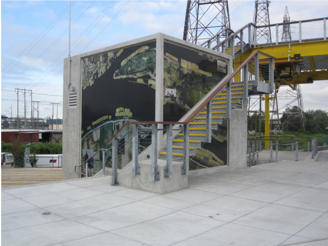
Public Art on the Control Building
