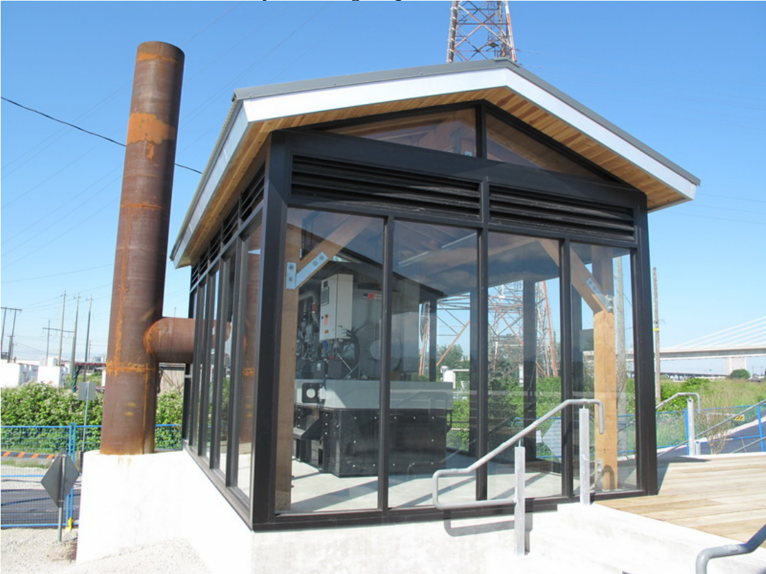
Completed Back-up Generator Building
