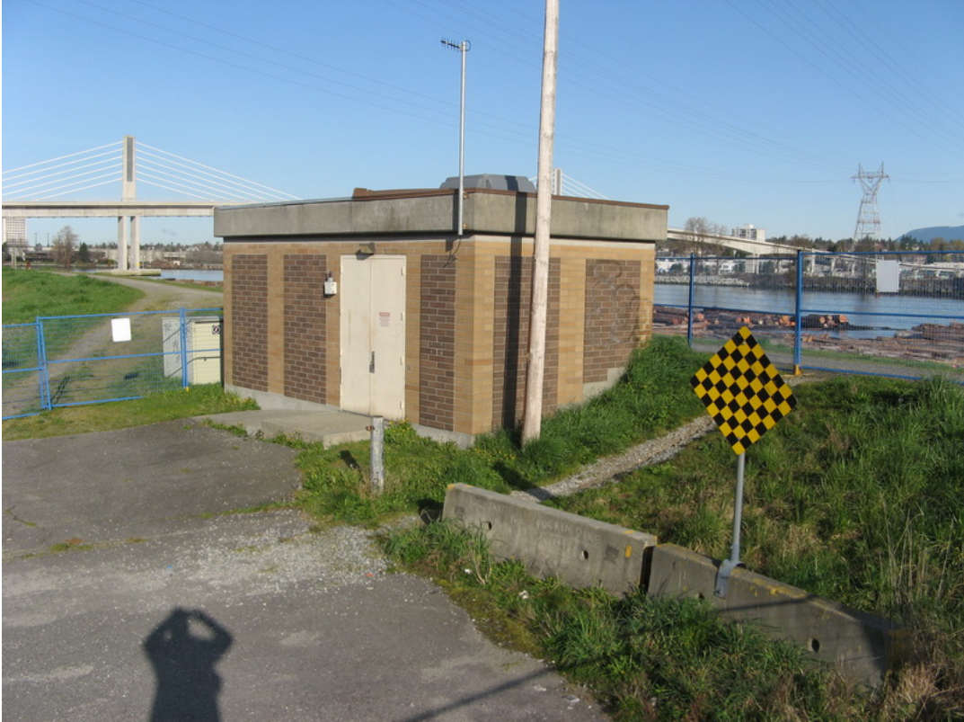
Original Pump Station
