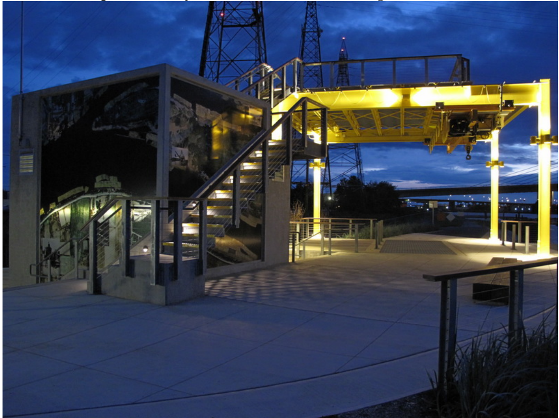
Completed Pump Station
