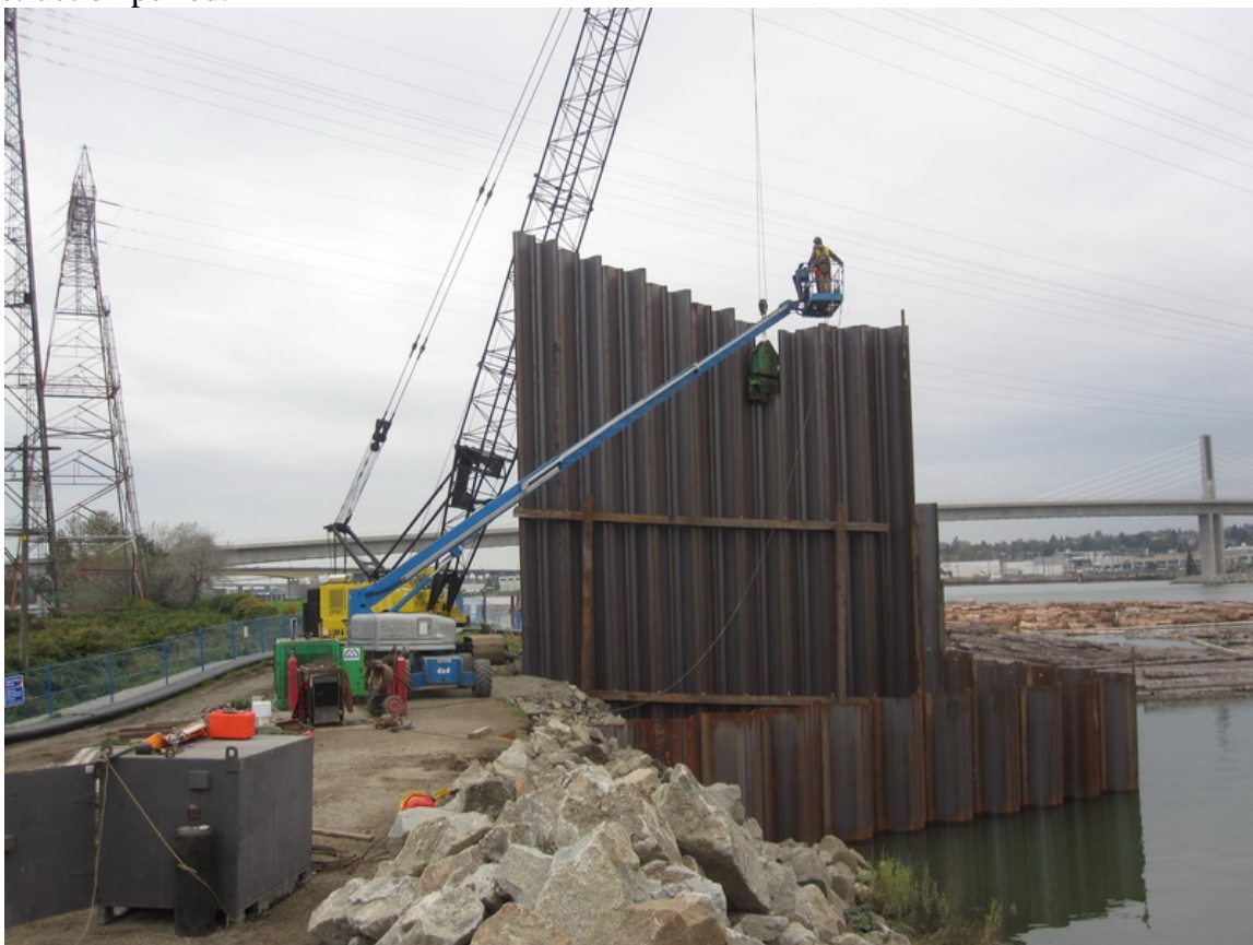
Cofferdam construction
