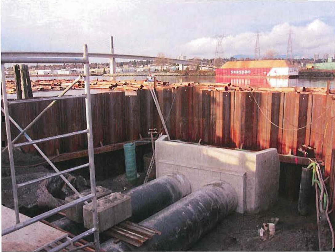
Gravity Discharge Pipes and Headwall
