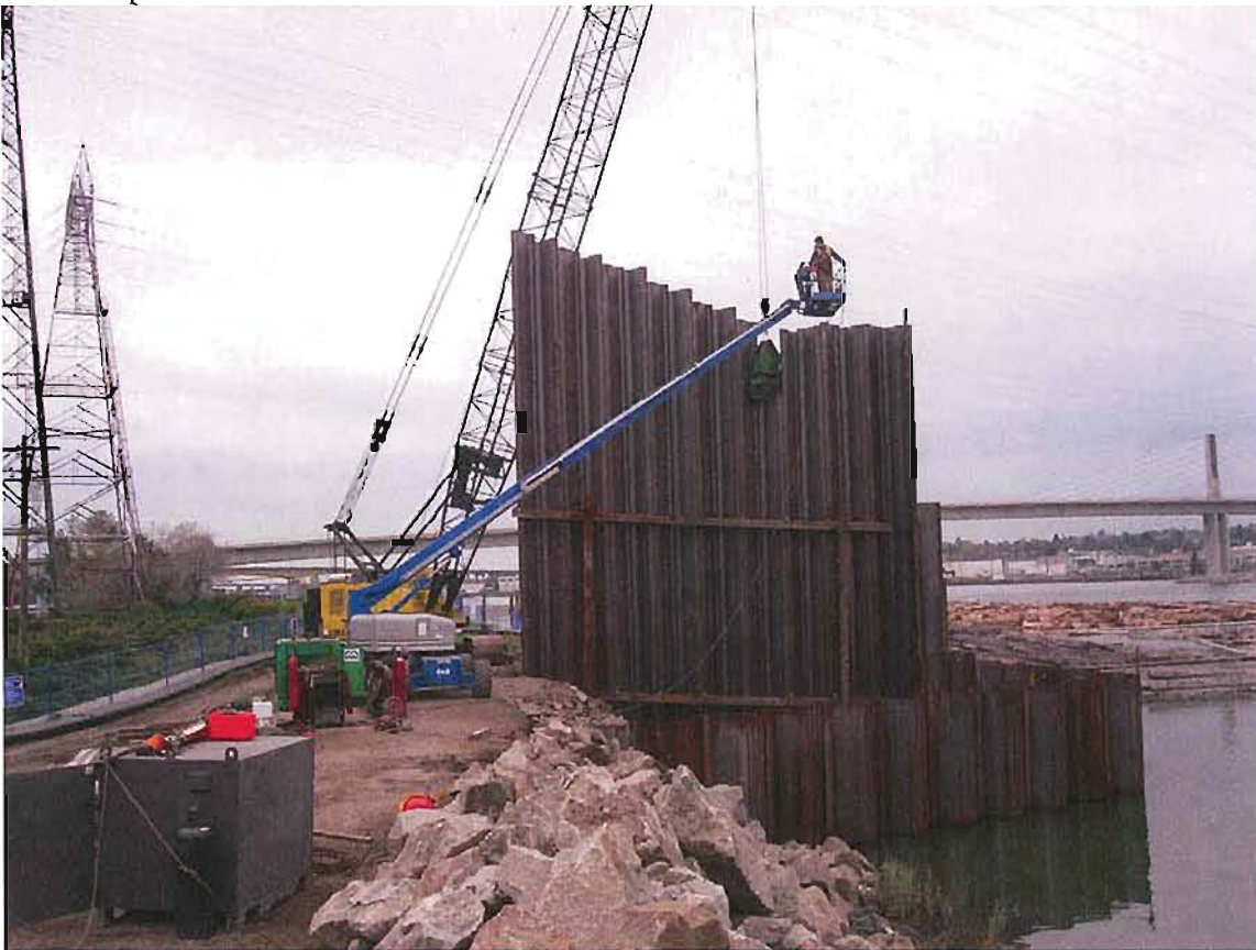
Cofferdam construction
