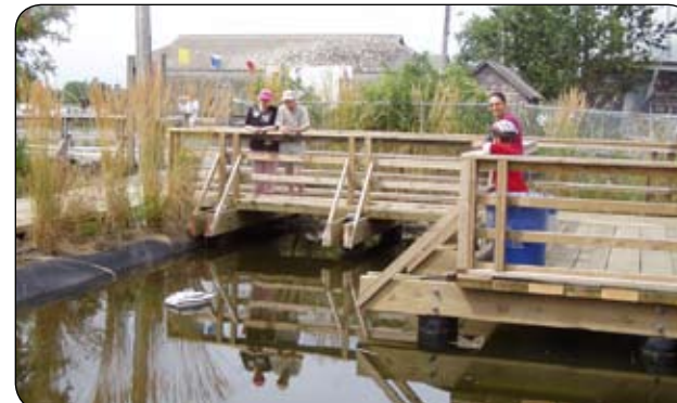
Britannia Heritage Shipyards: 'historic zone' stilt house restoration
