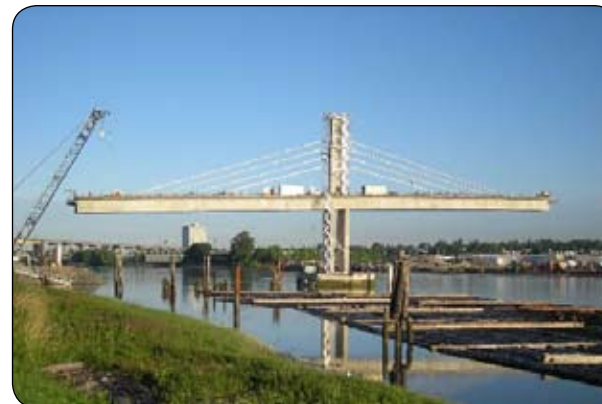
New North Arm Bridge for CanadaLine
