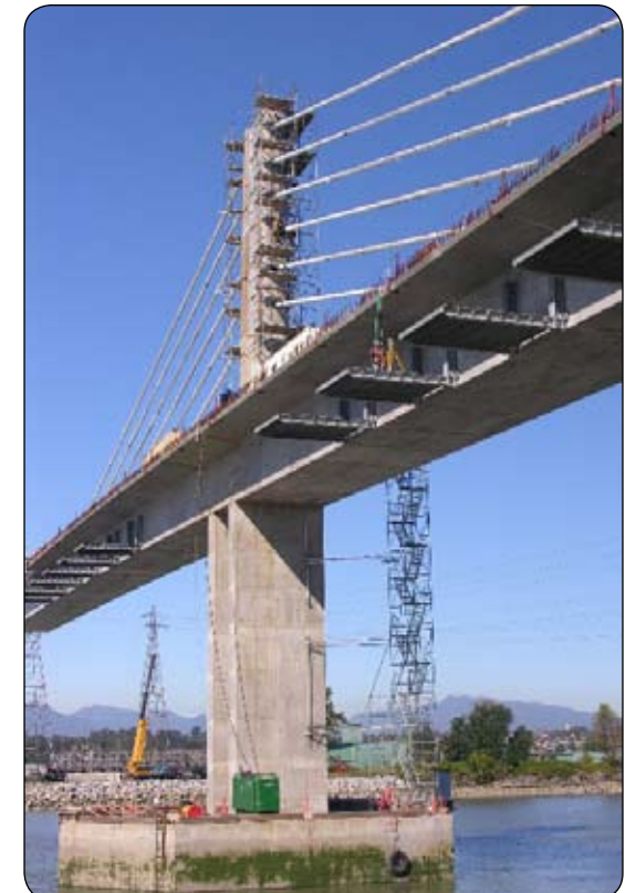
Canada Line: North Arm bridge and bike lane construction
