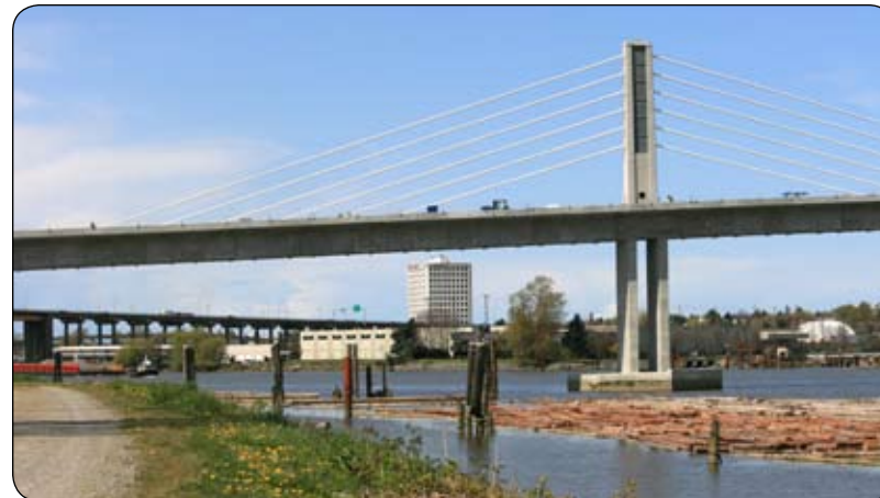
View of CanadaLine bridge from River Road and Shell Road
