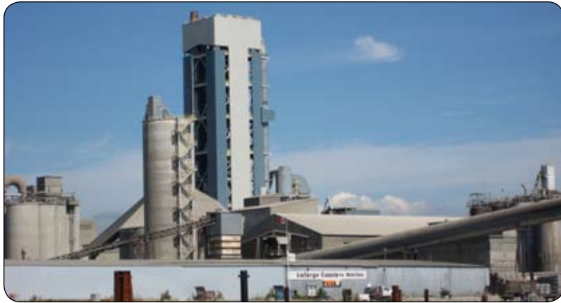
Concrete manufacturing facility
