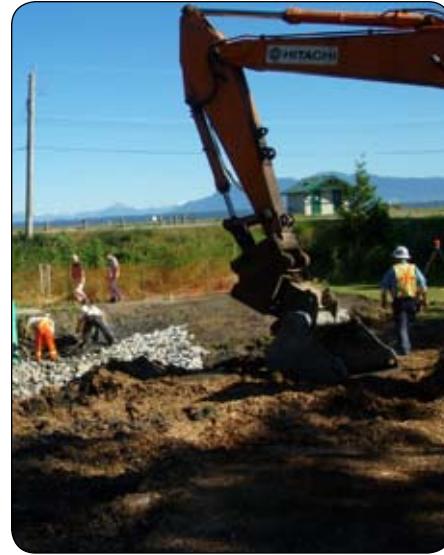
Terra Nova Rural Park: Slough construction
