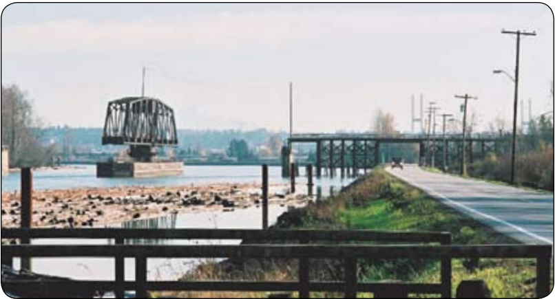
River Road: view east towards rail bridge
