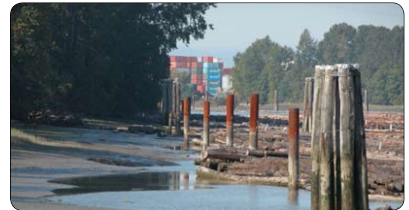
View from No. 7 Road Pier looking west
