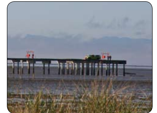
YVR maintenance crews on jetty
