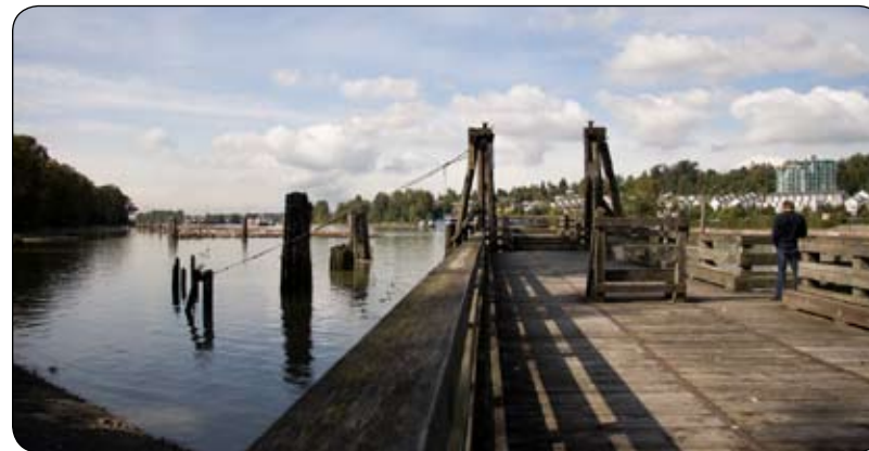
No. 7 Road Pier
