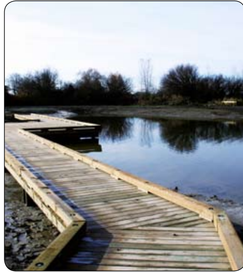
Terra Nova Rural Park: Slough construction
