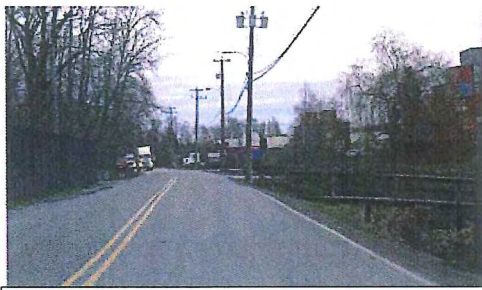
River Road Looking East (west of No. 7 Road). Narrow Road, Minimal Shoulder, Steep Ditch to the Right. Fence near Road to the Left
