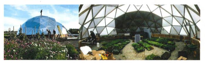
During the fall of 2018 we began the construction of our geodesic passive solar dome. This is a prefabricated kit that provides greenhouse space that can facilitate year round production without the input of fossil fuel energy. This greenhouse does not require any supplemental energy input. It captures solar radiation and relies on the design to facilitate efficient year-round heating and cooling.
