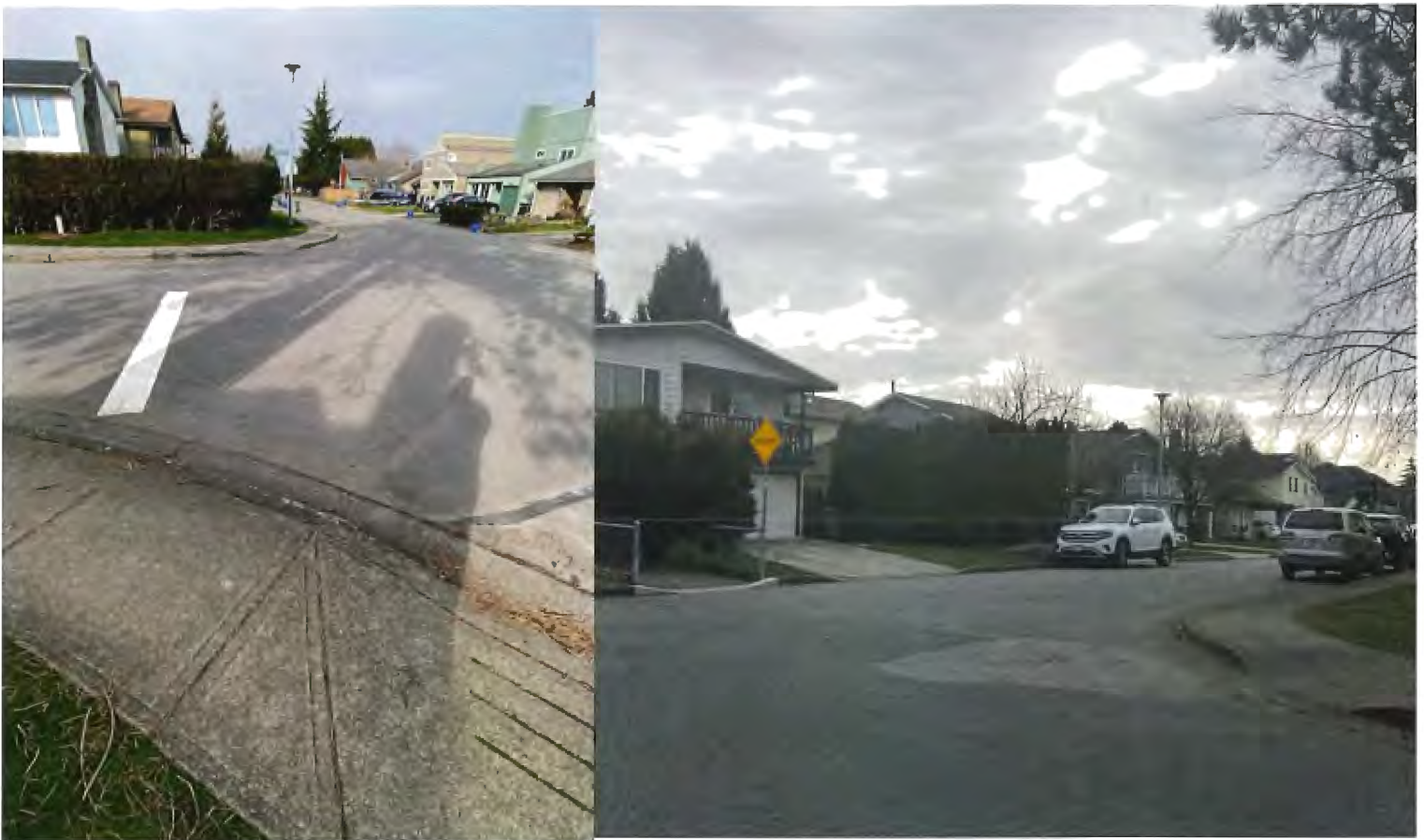
Fig. 5 - Sidewalk and walkway at the intersection of Hollymount Gt and Hollymount Dr, leading to the pedestrian walkway and McKinney Elementary School.
