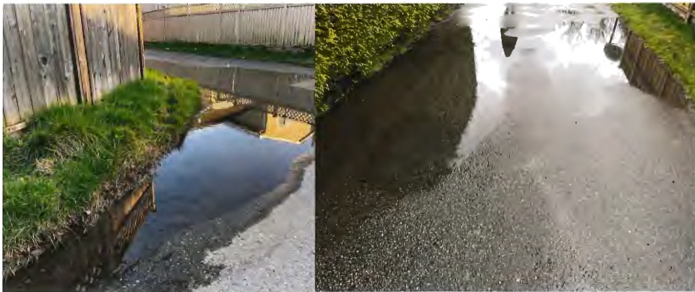
Fig. 3 – Laneway at the rear of the subject property, parallel to Railway Ave.
