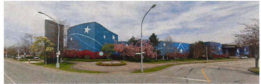
5 VIEW OF THE EXISTING THEATRE FROM THE CORNER OF ENTERTAINMENT BLVD & STEVESTON HWY SCALE: NTS
