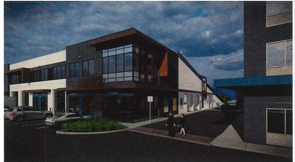
2 VIEW OF SOUTHWEST CORNER OF COMMERCIAL BUILDING SCALE: N.T.S.
