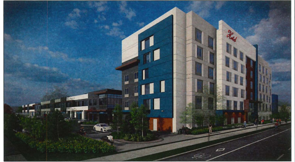
2 VIEW OF SOUTHWEST CORNER SCALE: N.T.S.
