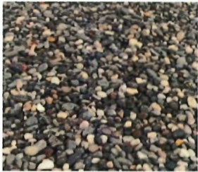
EPDM ROOF MEMBRANE ROCK BALLAST
