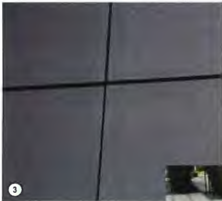
3 POWDER COATED ALUMINUM PANEL CHARCOAL COLOUR TYPICAL RECESSED CLADDING DURASTAR CHARCOAL GRAY #UC143865 (PPG)
