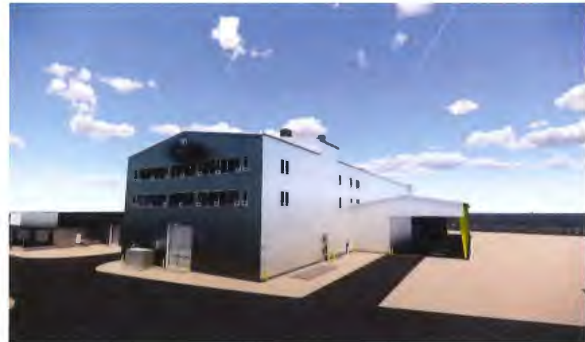
New machine shop showing attached covered storage area
