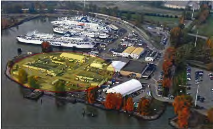
Existing FMU Facility Aerial (Highlighted Demolition Area)
