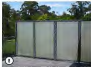
8 FROSTED GLASS PRIVACY SCREEN BETWEEN BALCONIES
