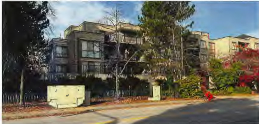
4 story apartment - flat roof
