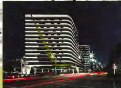
CASCADE CITY (BUILT)
