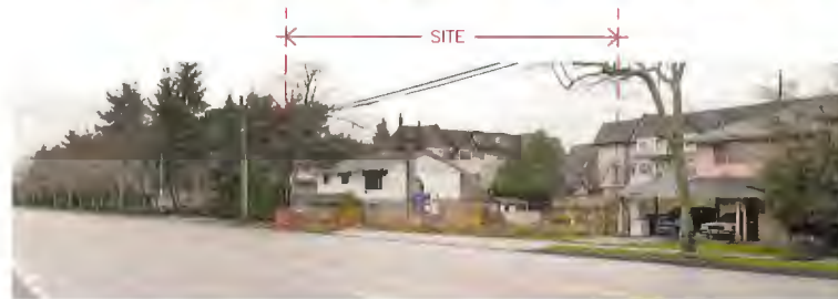
SITE VIEW ACROSS NO 1 ROAD
