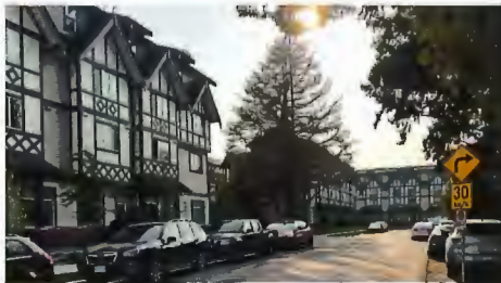
D EXISTING FOUR-STOREY TOWNHOUSES (SPIRES I)
