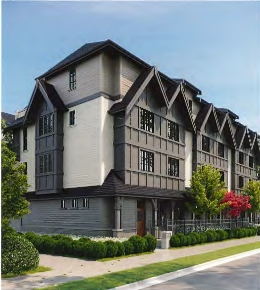
BUILDING 3 LOOKING NORTH
