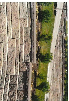
Allian block retaining wall
