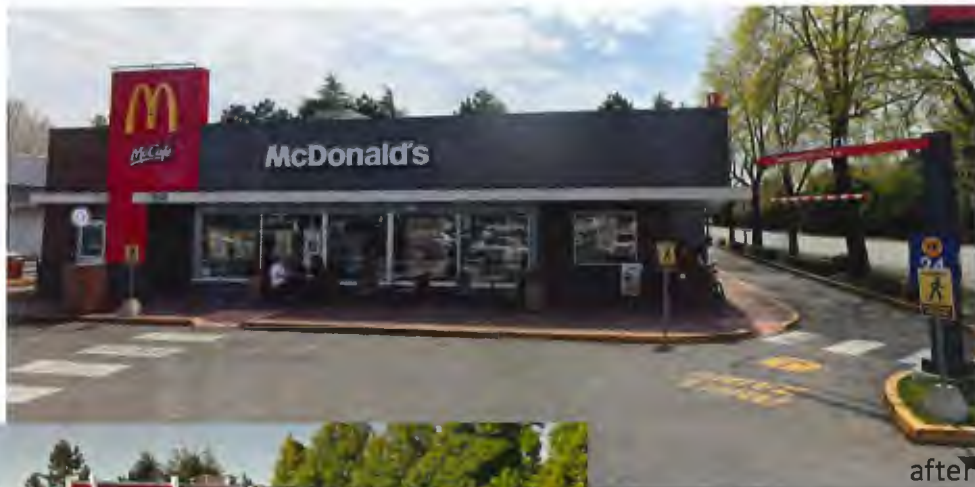
View of north side after
