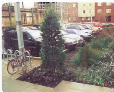
Permeable landscaped strip/swale collects run-off water from the paved parking lot allowing natural absorption of rain water and contribute to irrigation.
