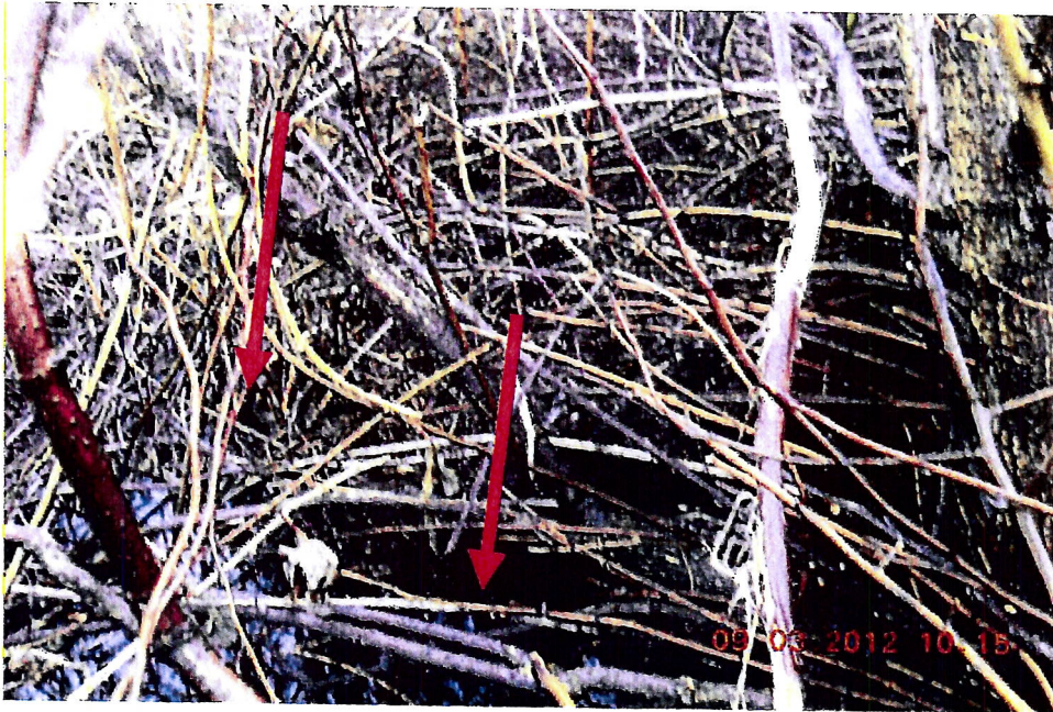
Photograph 11 Heavily Vegetated Northern Drainage Swale.
