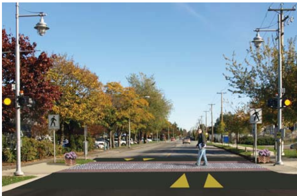
Figure 6: Raised Crosswalk on Moncton St at Easthope Ave (Motorist Perspective)
