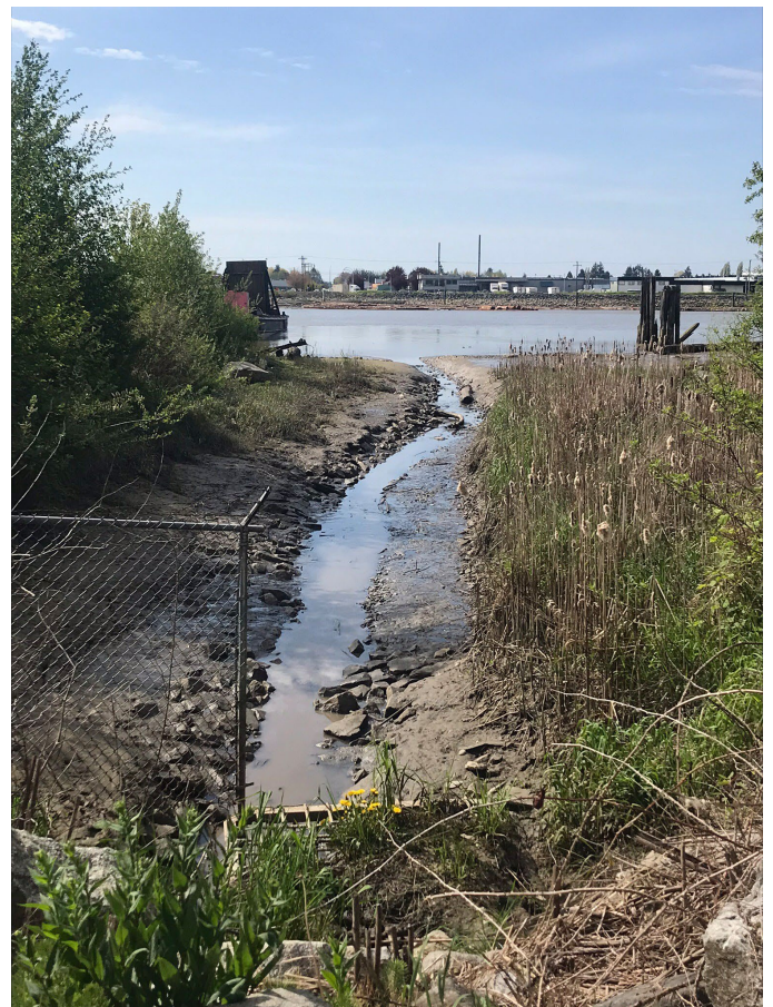
Oil sheen on water discharging from a stormwater outfall on Mitchell Island.
