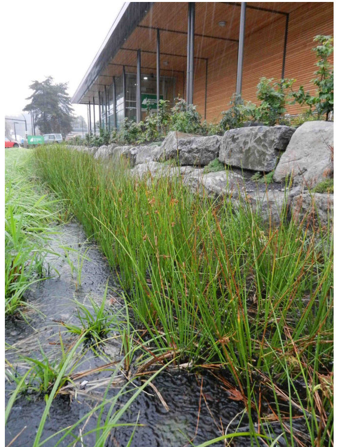
Example of bio-infiltration.
