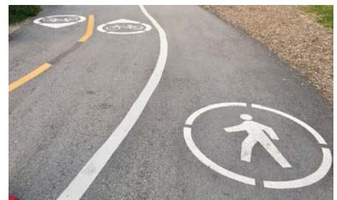
INSPIRATION: A painted line and symbols can be used to define uses where space is limited.
