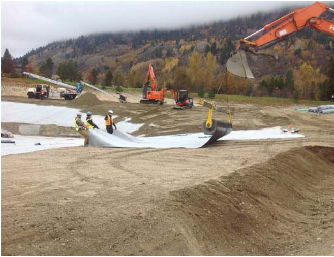
EXAMPLE: Bentonite liner being rolled out.
