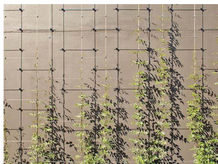
INSPIRATION: In the long-term, the grandstand could be upgraded and better integrated within the park. The structure could become an art or green canvas, interfacing with the Arts & Culture district.
