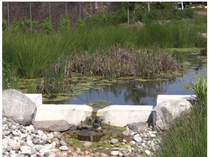
EXAMPLE: Completed channel.
