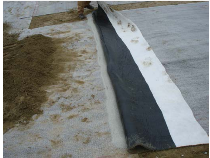
EXAMPLE: Bentonite applied to seal lap joints.
