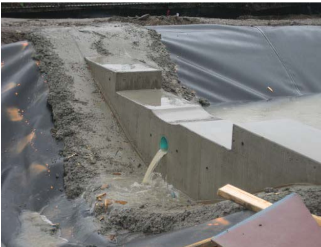
EXAMPLE: Weir structure for pond transition.
