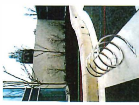
BOARD BIKE RACKS WILL BE FROM DOBRA DESIGNS; BLACK POWDERCOAT SURFACE MOUNT USING TAMPER PROOF HARDWARE
