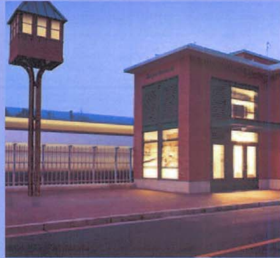
The new Columbia Street Pump Station helps reduce combined sewer overflows.
