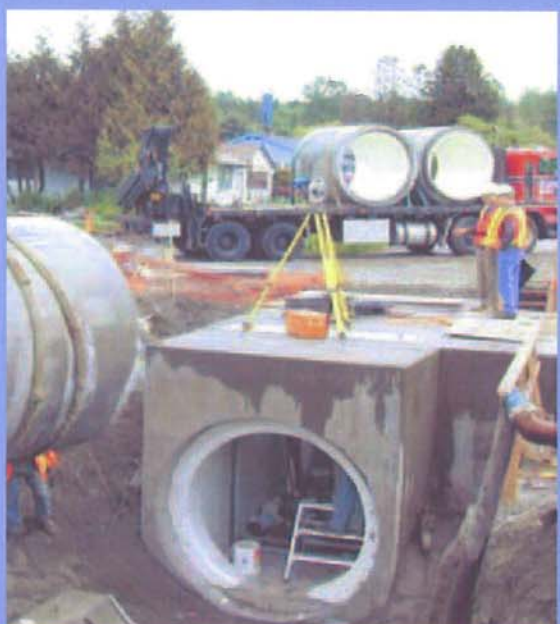
Installing Metro Vancouver trunk sewers, South Surrey.
