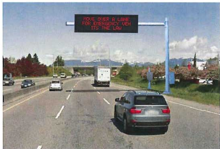
Figure 3: Rendering of Proposed DMS with Sample Message
