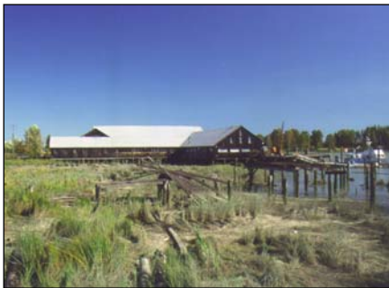
Britannia Heritage Shipyard and Cannery complex (c. 1889-1890)
