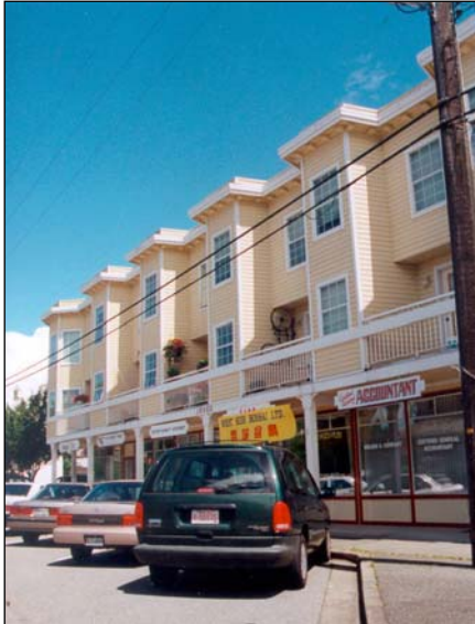
Mixed use commercial/residential on Chatham Street
