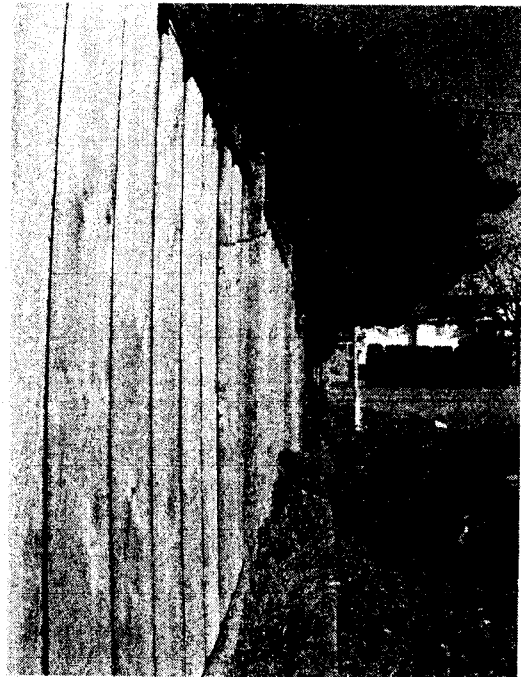
Photo showing the tree overhanging the fence into the subject property.
