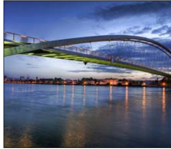
1. No. 2 Road Bridge
